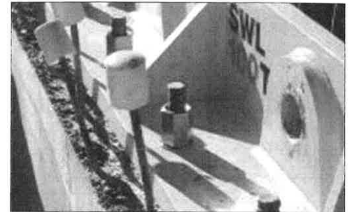
Reidbar™ continuous threaded reinforcing can be used to lift any size concrete element.
