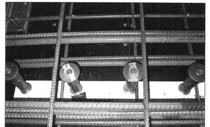
Reidbar™ Inserts™ used with ReidBox™ to simplify installation of floor to wall connections.
