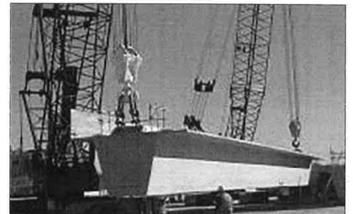
Reidbar™ was used as a designed lifting system to lift 200 Tonne Bridge Beams on the Kwinana Freeway Perth WA project utilising reusable lifting plates fastened with Reidbar™ nuts.
